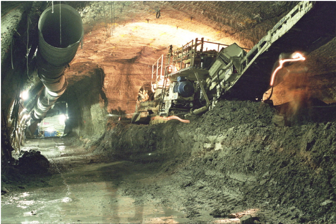
Photo 2 Macquarie Park Station – Concourse Cavern
