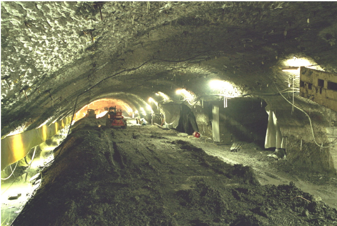
Photo 1 Macquarie Park Station – Platform Cavern, top heading
