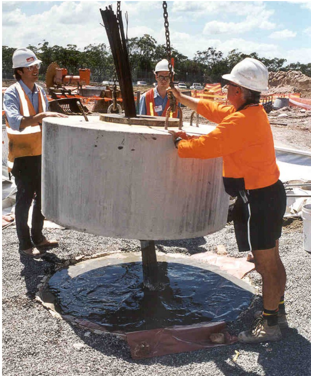
Figure 3 Positioning of reinforced concrete plate onto prepared ground surface.
