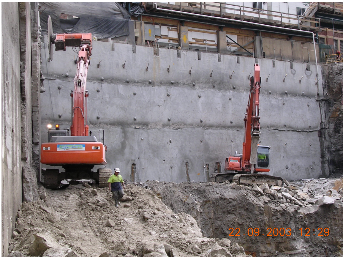
Photo 1: Partly excavated basement adjacent to George Street, Sydney
