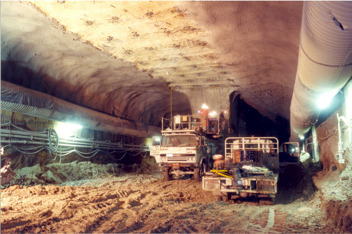
Photo 1 Excavation of Upper Deck of Piggy Back Tunnel
