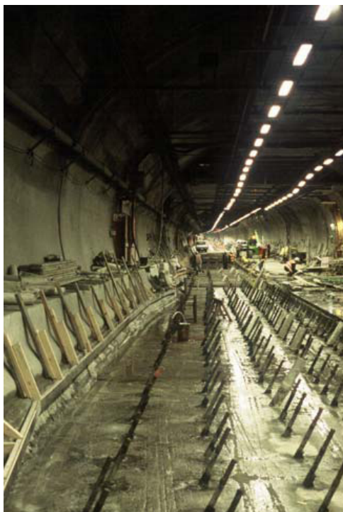
Photo 1 Drilling and installation of anchors.
